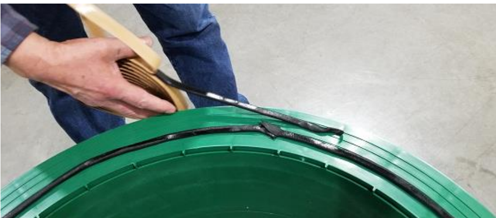
Form a second full ring of butyl. Flip the TAR over and press it firmly to the septic tank surface. Butyl should be minimum 3/8", butyl ends should be kneaded together
